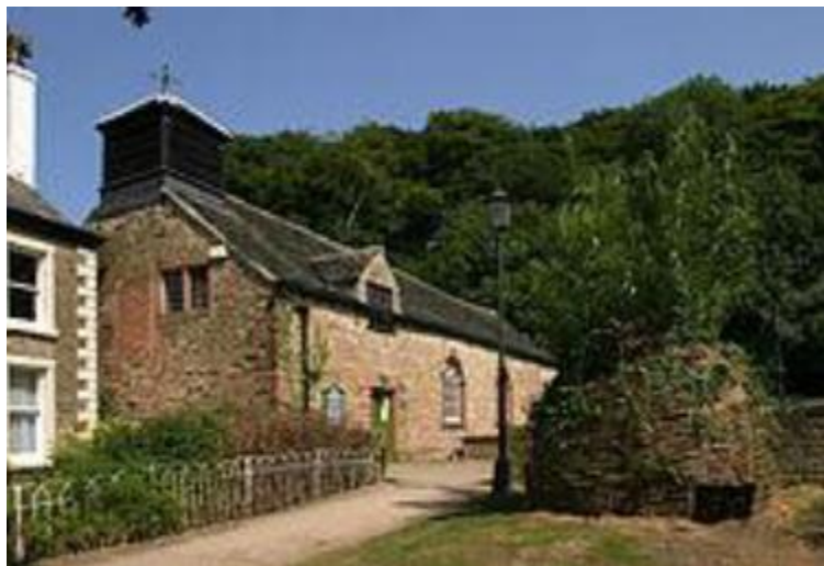
The west end of the chapel with the timber bell-cote
